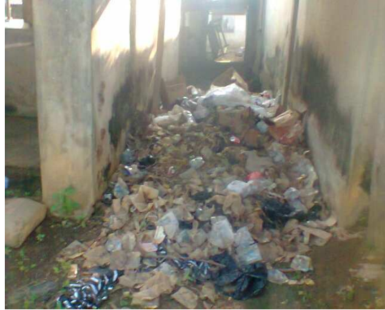
Fig 11: Improper disposal of waste between two slaughter slabs
